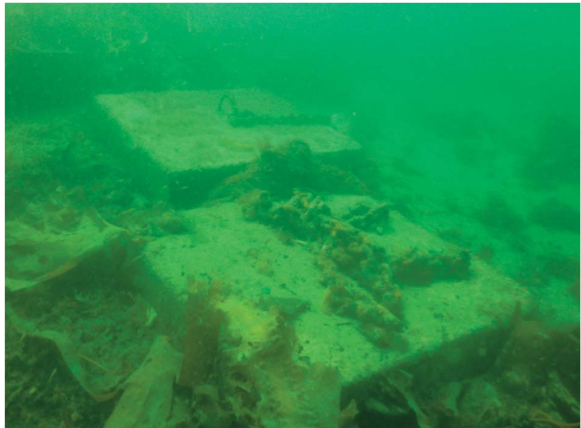
Plate B14: Mooring blocks identified during diver survey
